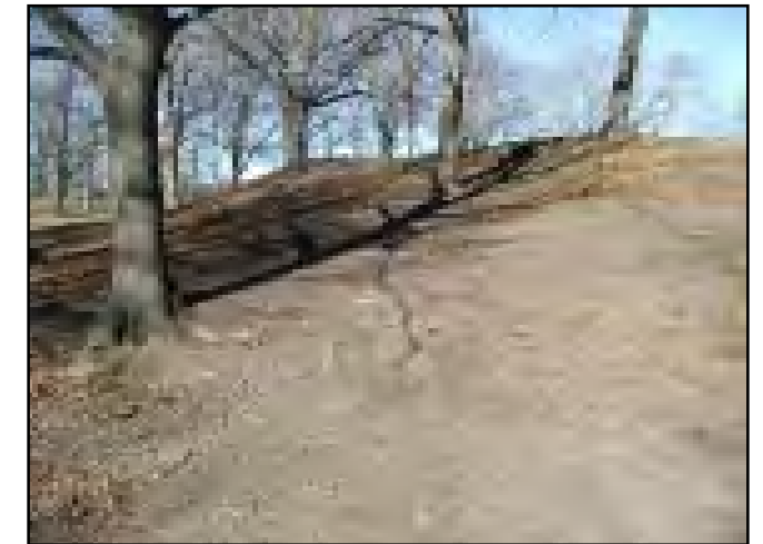
General area of erosion at the basketball court in Branch Brook Park. Heavy foot traffic in this area has trampled any vegetation that previously existed.
