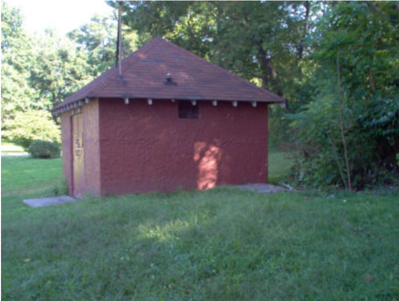
Photo 461 View of the Pump House from the southeast showing hip roof and over-hanging eaves.
