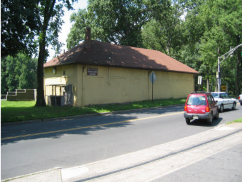
Photo 414 Overall view of the senior citizens center; note that all the windows on this façade have been infilled.
