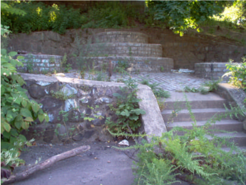
Photo 463 View of the Rock Structure from the east Branch Brook Lake walking path, showing the 3 stone structures which provide access to the sewer system.
