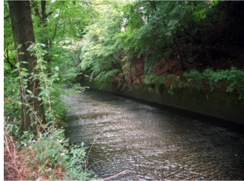
Photo 477 View looking east of North Branch Brook Park Drive Bridge showing steep south embankment and heavy tree and plant growth on both sides.
