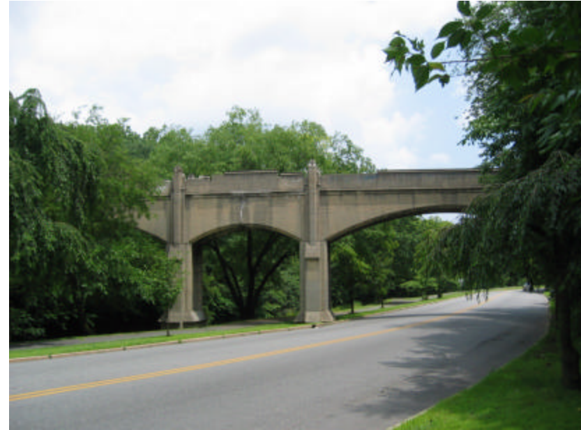
Photo 326 View east towards the bridge; note the difference in the size of the arches and the overall condition of the parapet wall.
