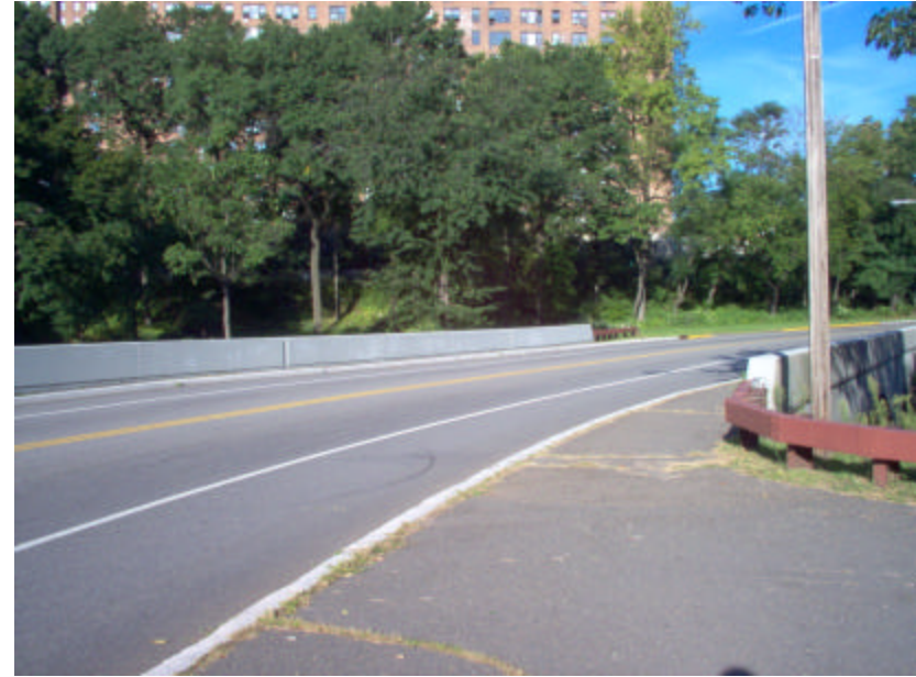
Photo 456 View of South Branch Brook Drive Bridge roadway from the east; note the concrete curbs and the single asphalt-paved sidewalk.
