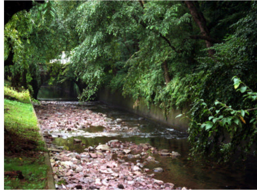
Photo 483 View looking east toward Summer Avenue Bridge showing accumulations of eroded stone; note the dense growth on the south embankment and the grassy sitting area on the north.
