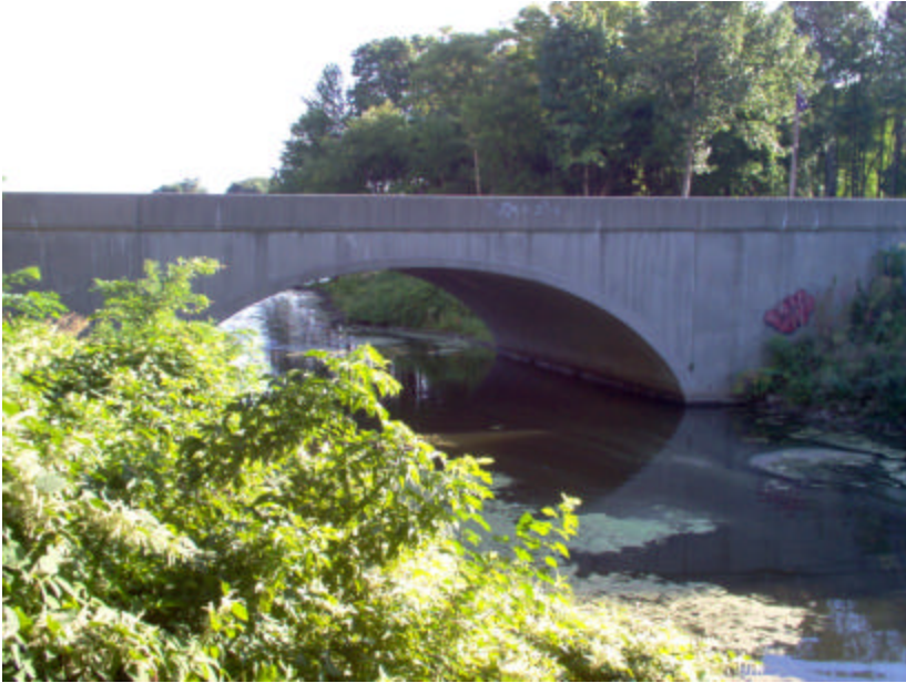
Photo 457 View of South Branch Brook Drive Bridge from the south.
