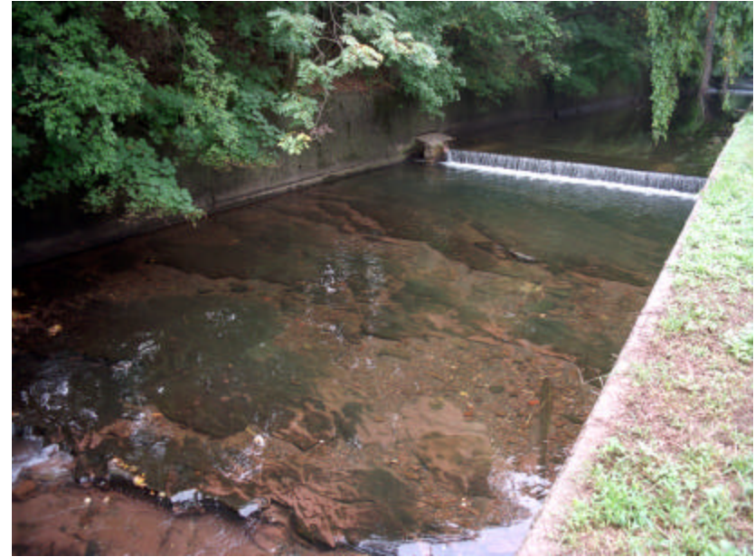
Photo 485 Detail of the natural stone channel bed and the concrete waterfall east of the Summer Avenue Bridge.
