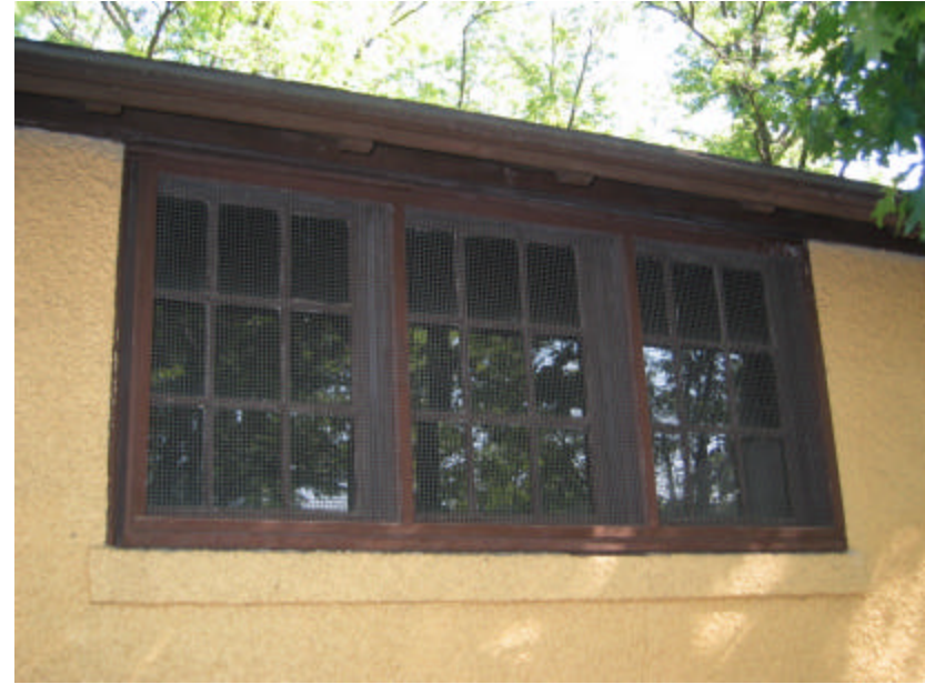
Photo 434 Three of the original wood sash hopper windows; note that they are covered by a metal screen.
