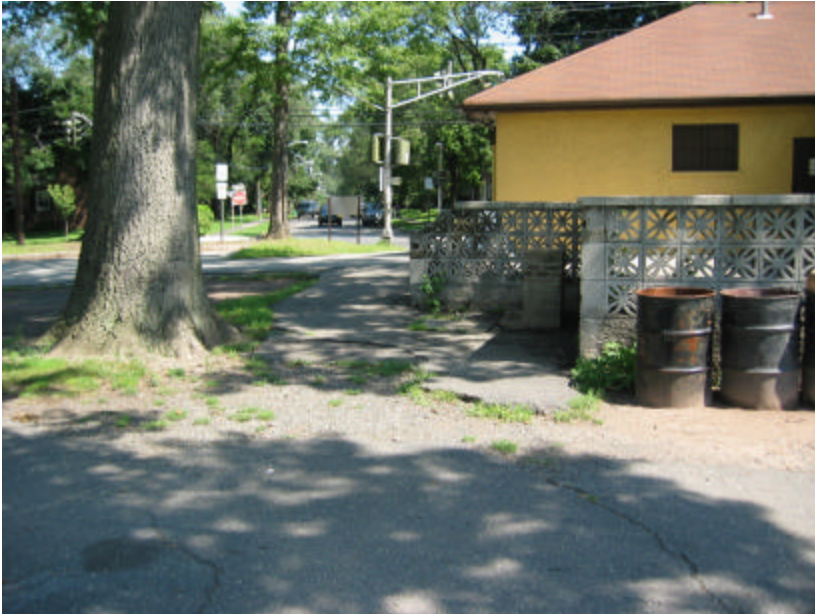
Photo 420 View north towards Belleville Avenue; note the buckled and cracked asphalt paving.
