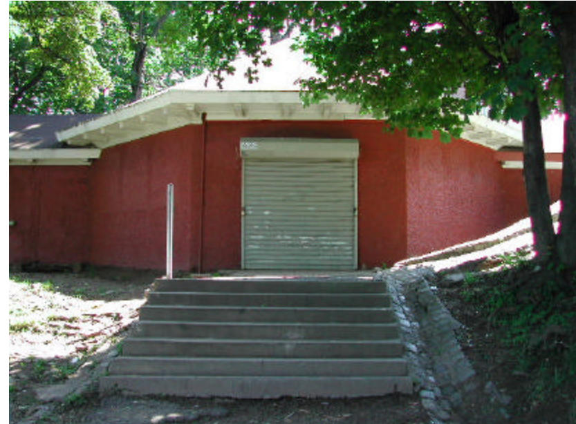
Photo 451 Detail of the west entry elevation as approached from the Middle Division ballfields; note the extensive erosion.
