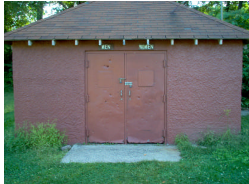
Photo 462 Detail of the south entry elevation showing painted pebble-texture finish; note the poor condition of door and shingles.
