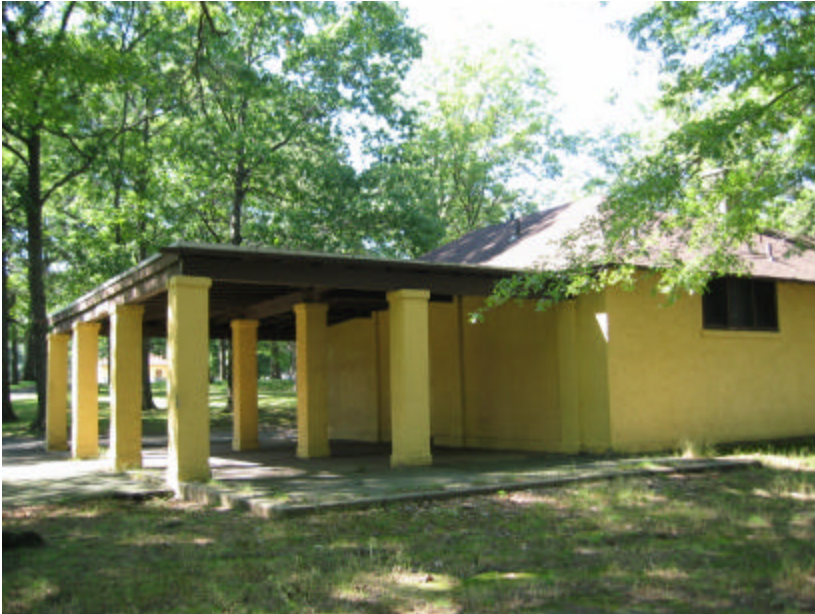
Photo 431 The covered veranda extending from the building's front façade; note the square columns.
