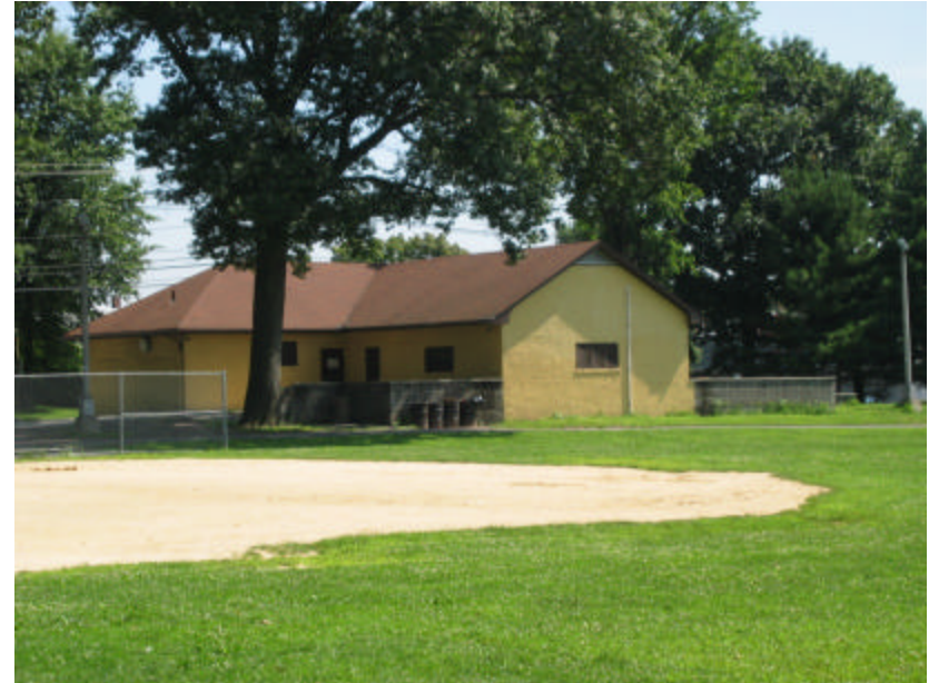
Photo 419 View northeast over the baseball field towards the senior citizens center; note that the site is flat.
