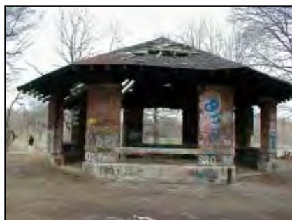
The Octagon Shelter (southeast face).
