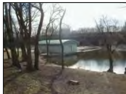
The Boat House, looking southwest across the lake (Interstate Route 280 in background).
