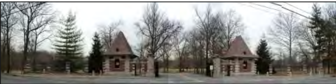
Formal “Ballantine Gateway”, looking west across Lake Street at Ballantine Parkway.
