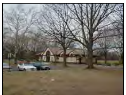
Branch Brook Park Visitors' Center, looking northwest from pedestrian entrance at Verona Avenue.
