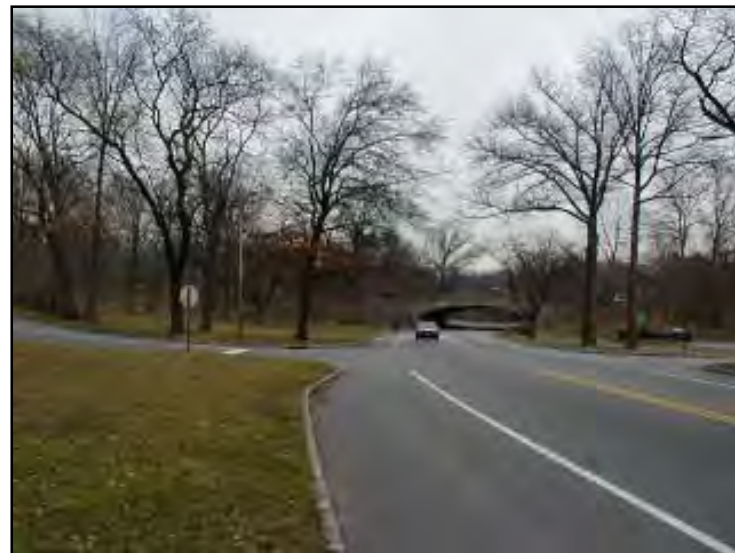
The Bloomfield Avenue Bridge, which separates the Middle from the Northern Division (view is toward the north from the Seniors' Center).
