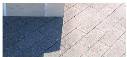
Top: Asphalt paving for pathways: standard primary path is 10' wide, standard secondary path is 8' wide. Cross slope path (do not crown) to allow for snow removal. Use standard NJDOT asphalt mix. Bottom: Asphalt block paving is Hanover asphalt block pavers, color matrix A80012, finish "Heavy Tudor"; size: 12" x 5" rectangle or 12" x 6" rectangle. Border paving areas with 12" wide rowlock course, while the field of pavers should be set in running-bond pattern.
